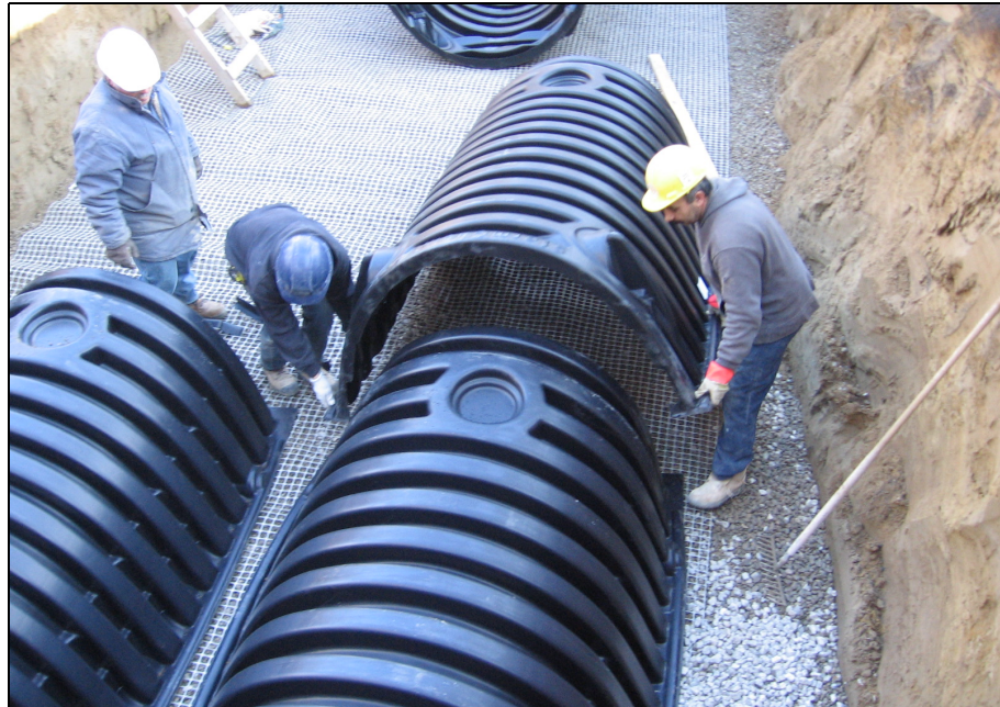
Figure 8.12 Installation of an underground stormwater storage chamber system
