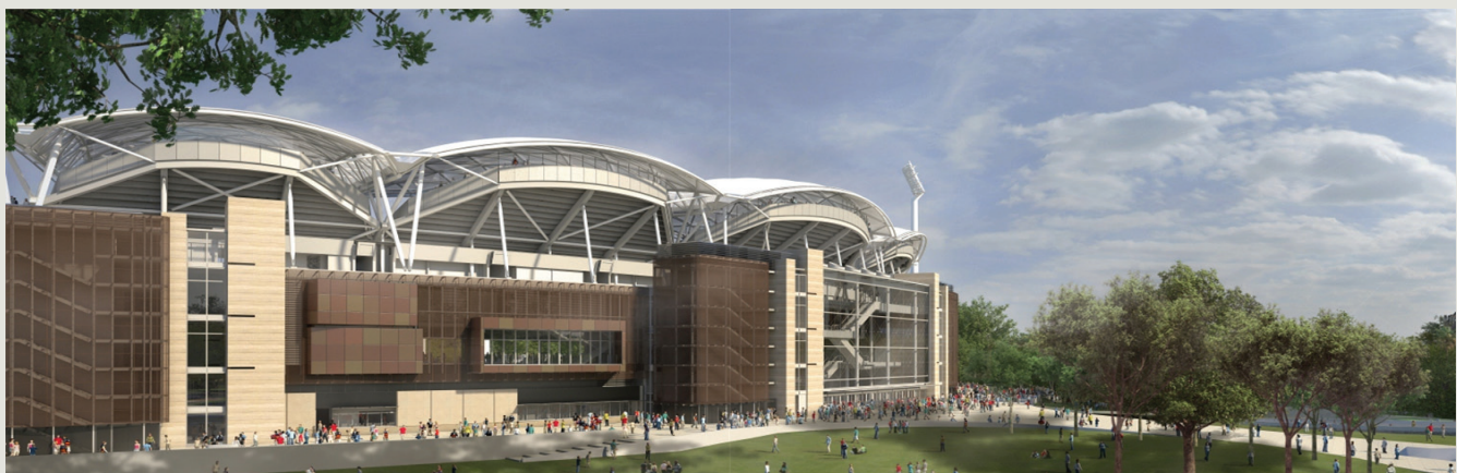
To develop the Adelaide Oval, multiple team members from a variety of disciplines needed to author and access project data. The team created a BIM execution plan to contractually establish terms and expectations.
