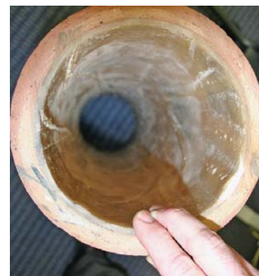
Vitrified clay pipe in St. Paul containing a plastic inner coating is the least of the worries of the St. Paul Public Works Department. Unreinforced concrete pipe installed in the 1920s takes priority for repair.
